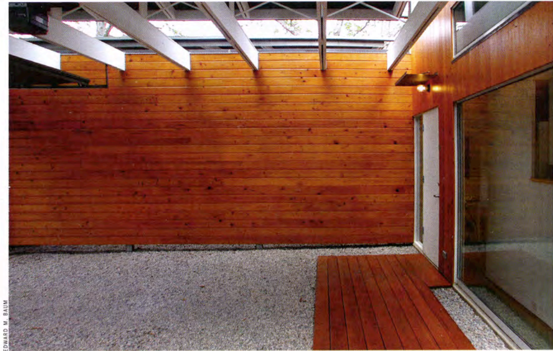
Above: The roof canopy of the auto courtyard is made up of a series of trusses. They are very rigid in the spanning direction; strength in the other direction is achieved by cross bracing using rigid electrical conduit as bracing material. Left: The forward bedroom is 12 by 14 feet (3.7 by 4.3 m), but the long glass wall onto the central courtyard makes it appear much larger. It also can be used as a home office, library, guest room, or other flexible space.
